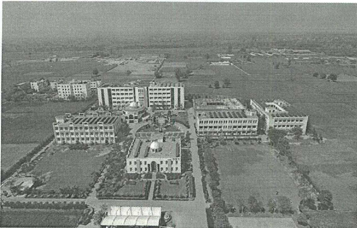
Figure 1. Panoramic view of the institute campus showing entrance-parking at the front
