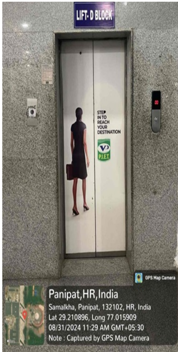
A picture of lift in D Block
