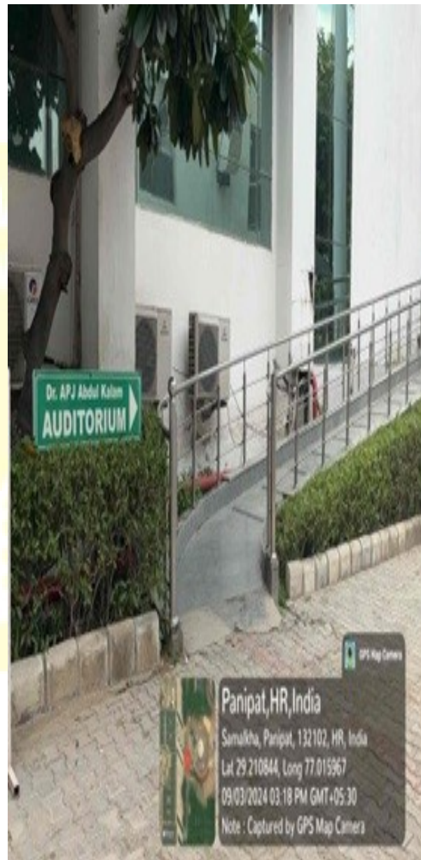
A picture of ramp near D Block
